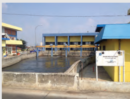
Figure 14.1 Tengah Pumping Station, Jakarta, Indonesia, refit completed in 2014, lifts water up from the Waduk Pluit lagoon.
