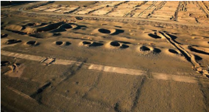
Figure 2.2 Access points of the vertical shafts in a Qanat system (Source: Iran Front Page).
