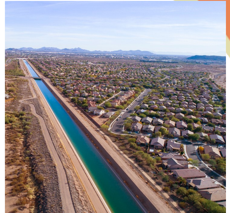
Central Arizona Project Canal
