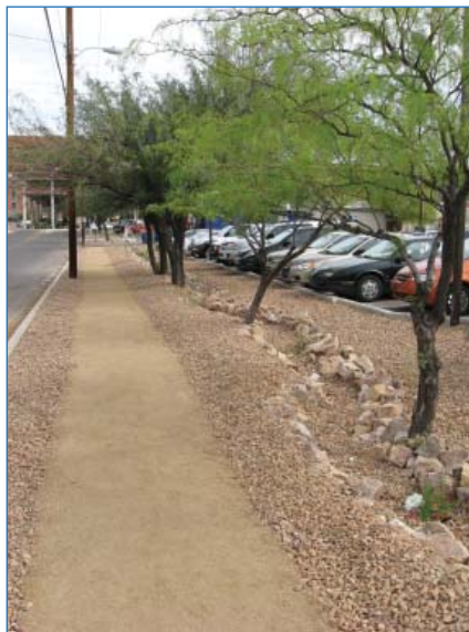
After: A long, thin swale was installed and additional trees and shrubs planted to capture and use runoff from the lot.
