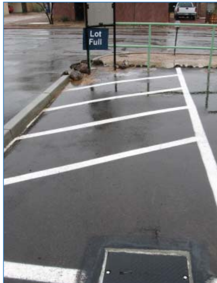
At this University of Arizona parking lot, an unused space happened to coincide with the lot's natural low point. The asphalt was removed and a bioretention basin installed. Note concrete header and curb stops. The basin's interior was terraced and shaped to distribute stormwater evenly. Overflow exits the back left corner and flows to the street.
