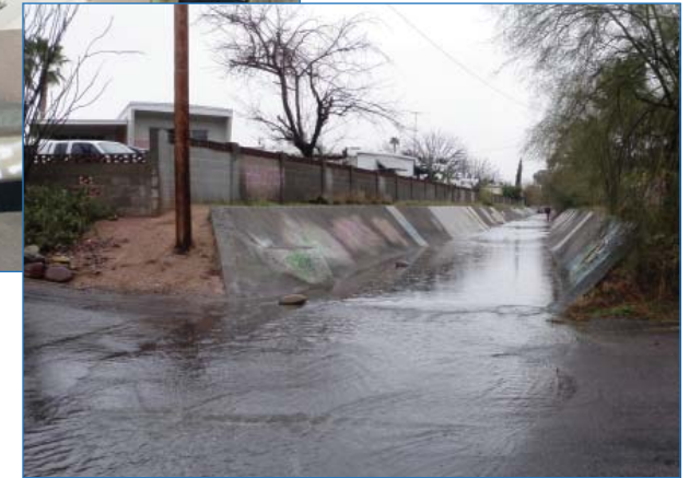
Grey infrastructure: Concrete channels, which have replaced natural washes, send stormwater quickly downstream.
