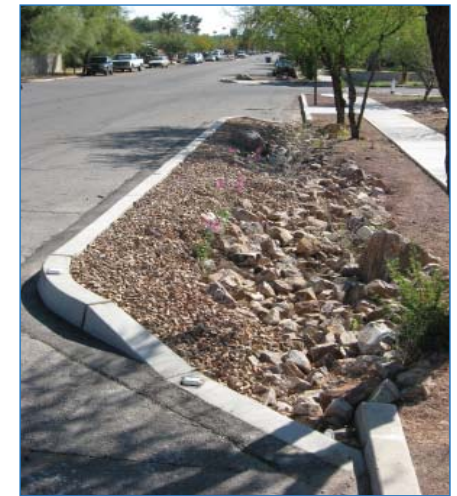
In this just-installed chicane, 4"-8" rip-rap is used in the channel where stormwater will flow rapidly, and 1" gravel covers upslope areas.
