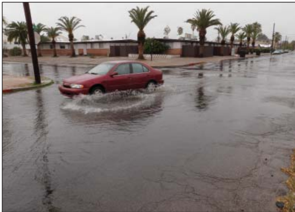
Many Southwestern streets are designed to convey stormwater.
