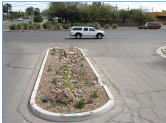
Median with curb cut
