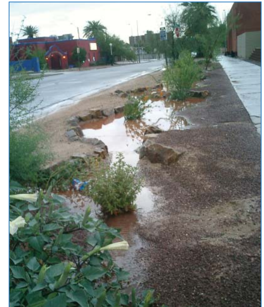
This series of basins collects stormwater from the adjacent sidewalk and businesses (without curb cut).
