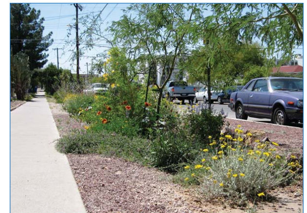
Soil, mulch and plants filter pollutants from stormwater. Some potential pollutants, like phosphorus, are taken up by plant roots as nutrients.
