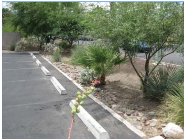
Bioretention basins, like this one between a restaurant parking lot and the street, capture and filter stormwater. Landscape area is graded below the level of the parking lot.
