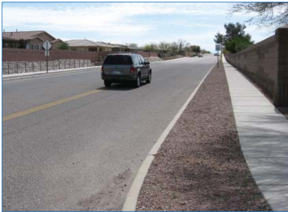
The ROW (for the purposes of this manual) is the strip of land between the street and private properties. This typical suburban ROW is devoid of vegetation.
