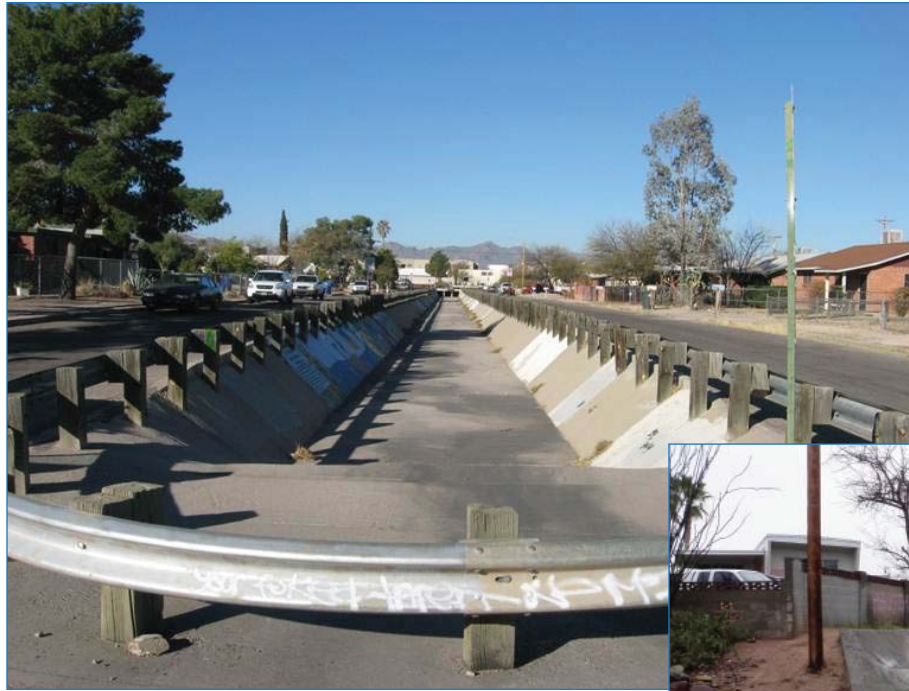
Grey infrastructure: Concrete channels, which have replaced natural washes, send stormwater quickly downstream.
