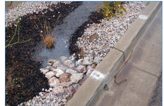
Curb cuts on a street in Flagstaff, AZ (left) and curb cores on a street in Tucson (right) are used to direct stormwater runoff from the street into basins before pollutants reach washes and rivers.
