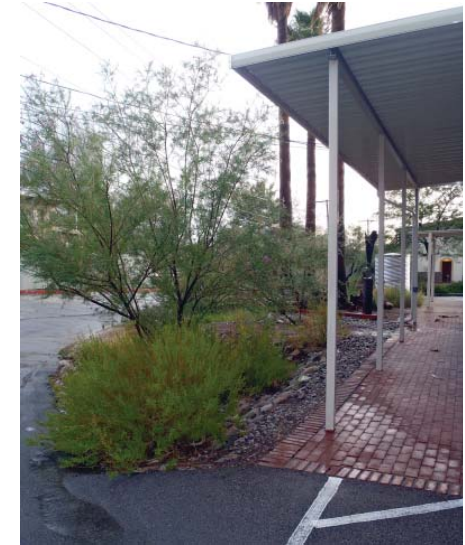
One year later, stormwater-fed native vegetation has grown to shade the parking lot and entrance. Note that basin slopes are lined with rock to reduce erosion.
