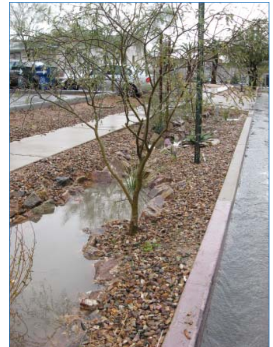
A velvet mesquite tree is planted on a terrace above the level of stormwater inundation at this GI site. This newly planted tree will eventually shade the sidewalk and street.
