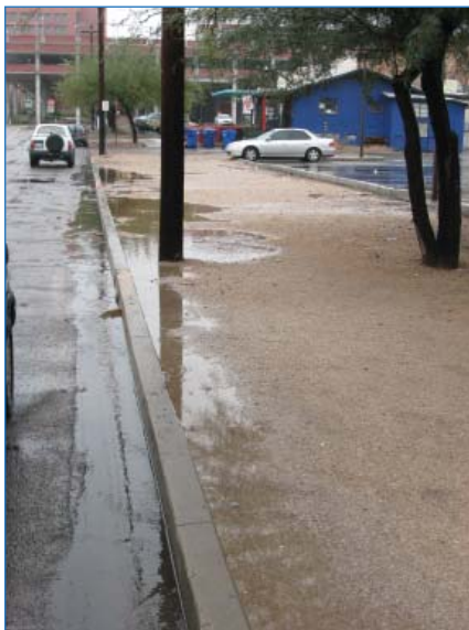
Before: At this University of Arizona (UA) parking lot, small curb cuts allowed stormwater to flow past existing trees onto the pedestrian area in the ROW, and then on to the street.
