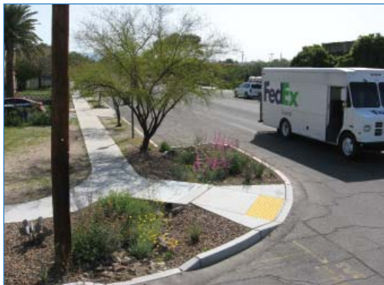
Chicane with curb cut
