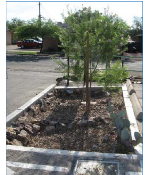
At this University of Arizona parking lot, an unused space happened to coincide with the lot's natural low point. The asphalt was removed and a bioretention basin installed. Note concrete header and curb stops. The basin's interior was terraced and shaped to distribute stormwater evenly. Overflow exits the back left corner and flows to the street.
