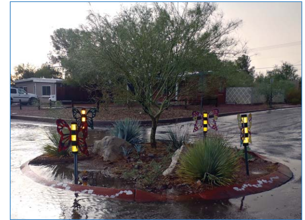
This traffic circle was designed to capture and retain the rain that falls on it.
