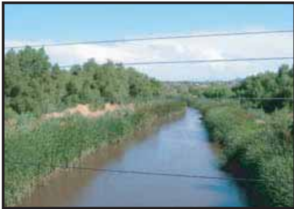
Effluent dominated Santa Cruz, view south from the Ina Road Bridge Tres Rios del Norte
