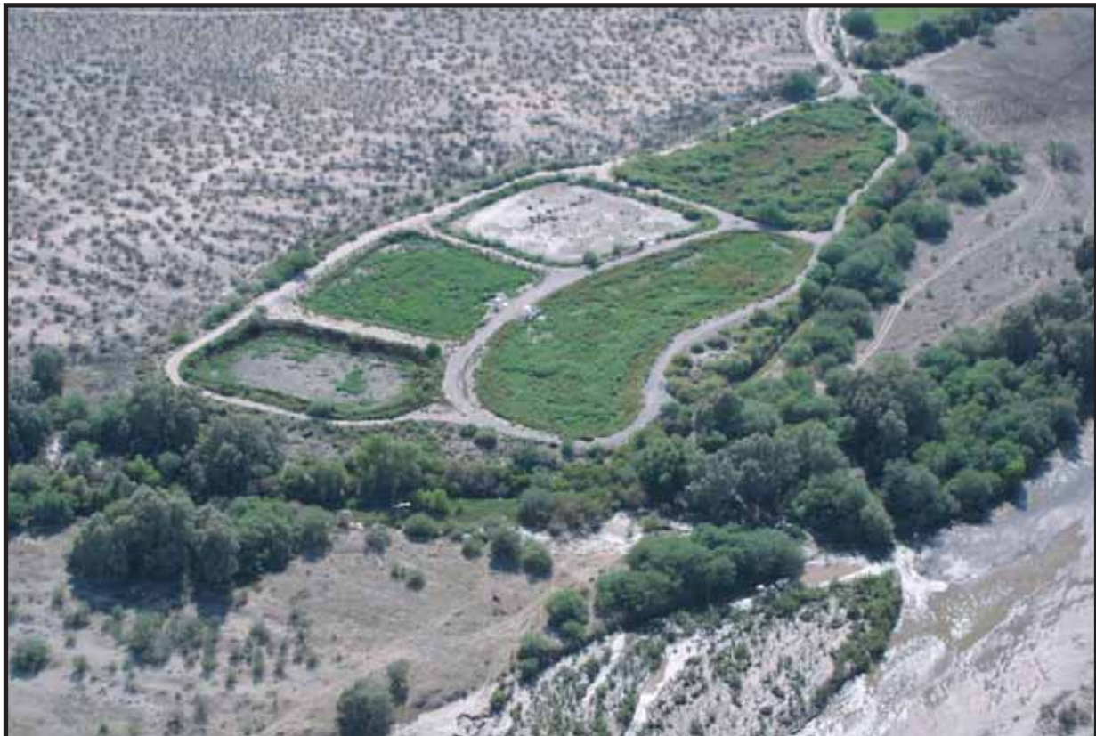
Aerial view of recharge facility and oxbow channel Marana High Plains
