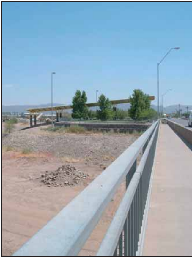
Park walkway Rio Salado Phoenix
