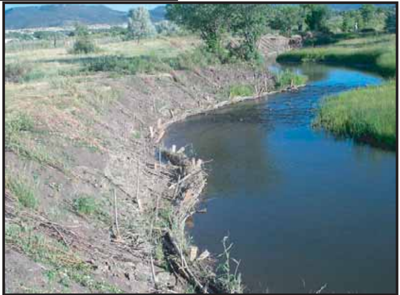
Bank stabilization Little Colorado River Enhancement Demonstration Project
