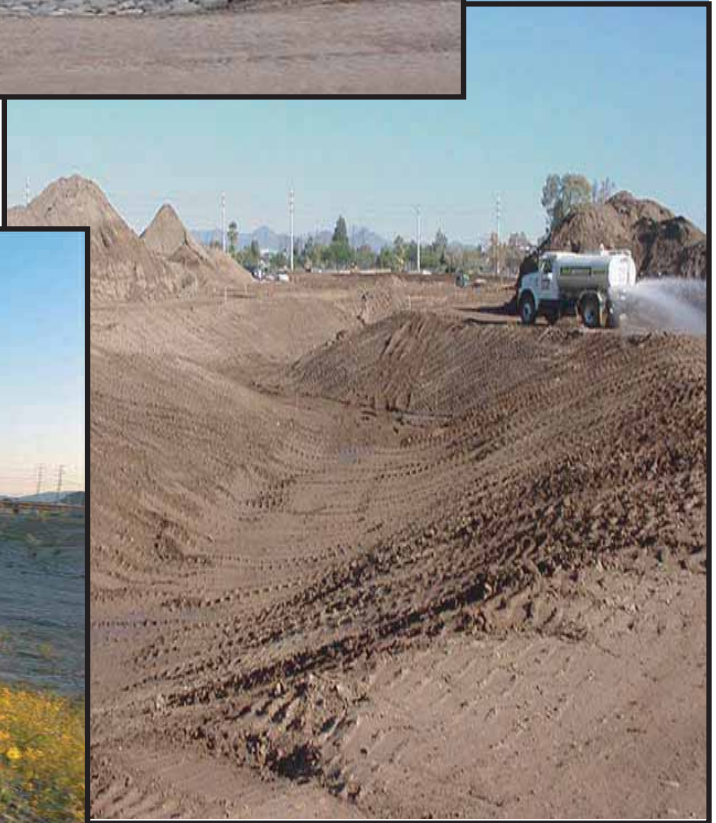
Indian Bend Wash Construction Rio Salado Tempe
