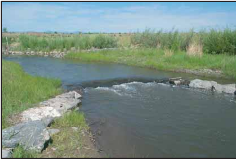
Construction Little Colorado River Enhancement Demonstration Project
