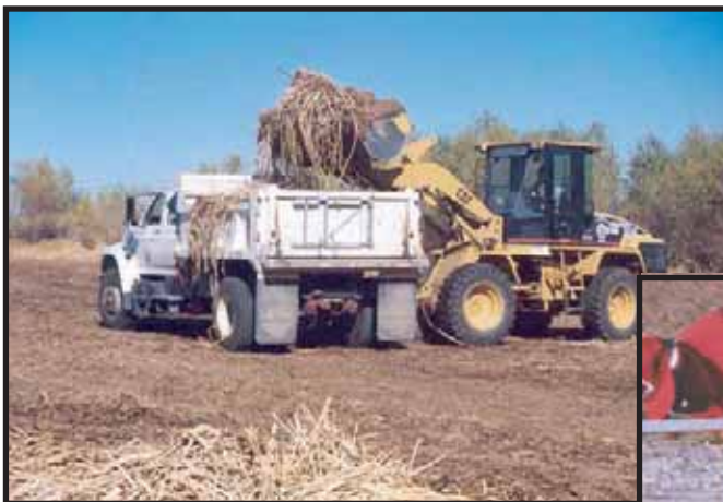
Operations- removing vegetation from infiltration basin Sweetwater Wetlands
