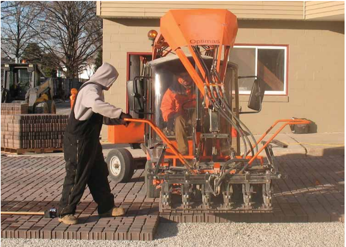
Installation of porous pavers at the Energy Exchange (November 2009).
