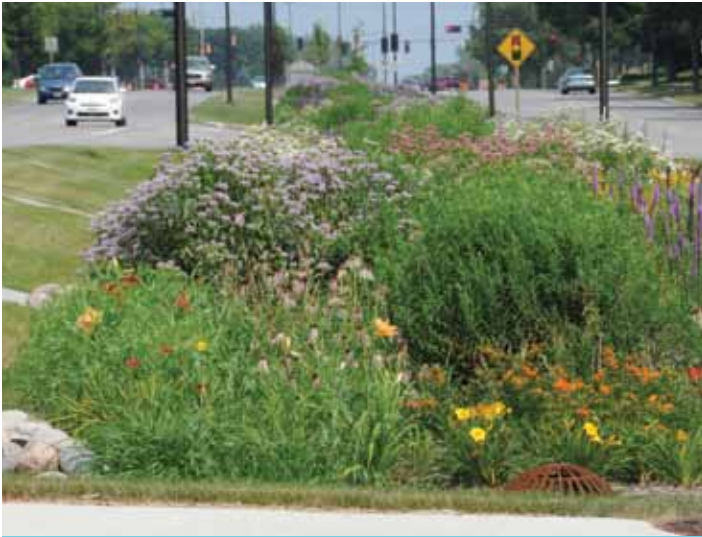
Bio-retention swales for stormwater treatment along Grange Avenue in the Village of Greendale.
