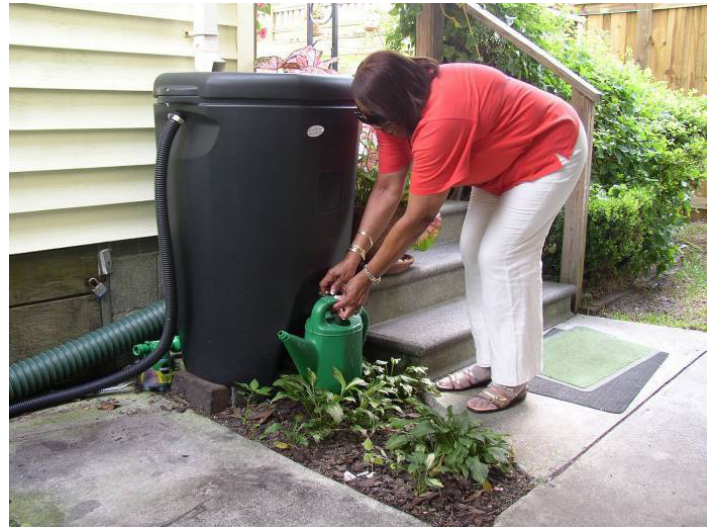
Figure 4. A manufactured rain barrel installed for watering flowerbeds
