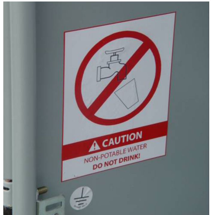
Figure 8. Stickers and decals remind users that untreated cistern water is not safe for drinking.
