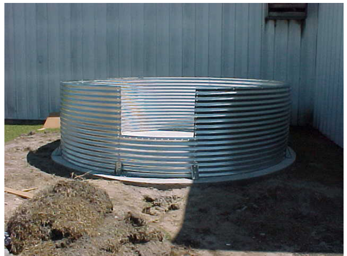
Figure 2. Metal rainwater cistern being assembled
