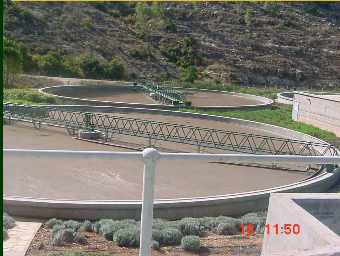
The Jerusalem wastewater treatment plant 2003
