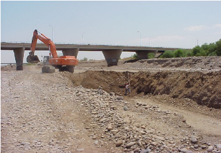
Construction of Low Flow Channel
