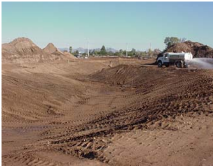
Indian Bend Wash Construction
