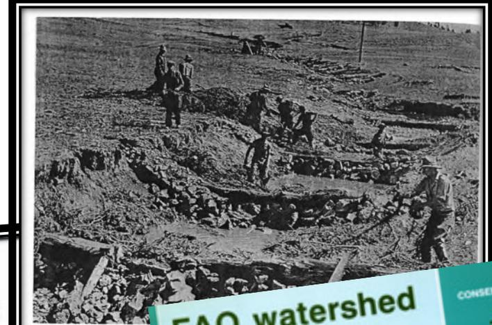
Figure 11. --In 1937, a gully by check dam in watershed shown. Since 1937 no further work has been done up about 90 per cent owned and lies abandoned started in the or loose rocks were. In the main gully, and many structures were built. data: Length of channel Number of check dams Average distance between check dams
