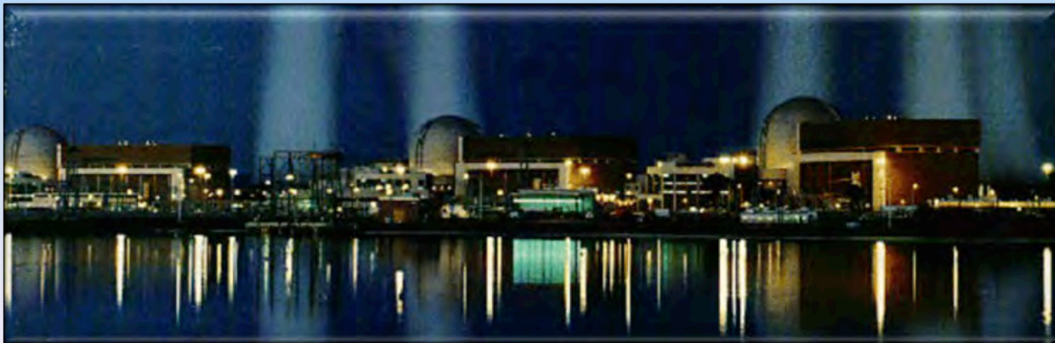
Palo Verde Nuclear Plant (APS)
