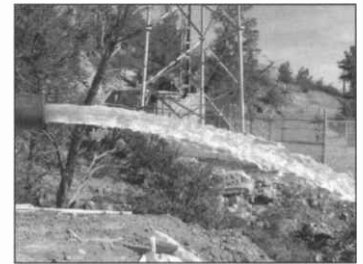
Pump test on a new well in Payson. Photo: Scott Stratton
