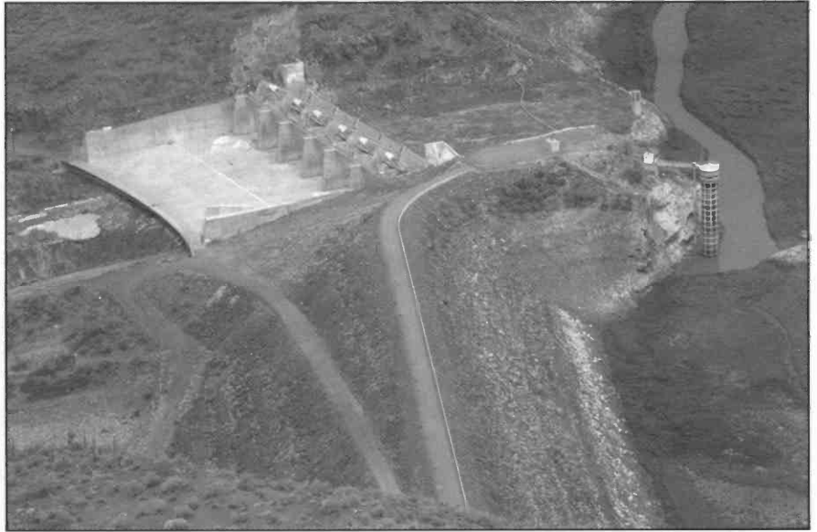
The effects of the ongoing drought dominate state water affairs, with officials hoping that El Niño will provide some much needed relief during February and March. Above is Horseshoe Dam, the upper most structure on the Verde River, now high and dry. Gone is Horseshoe Lake, with only a remnant of the Verde River now meandering in its old stream channel. Despite what the photo seems to show, water is still being released downstream of the dam. The outlet works are blocked from view by the hill in the bottom-left of the photo. The photo was taken in July, but the same conditions currently prevail. (Photo: Central Arizona Project, Phil Fortnam)
