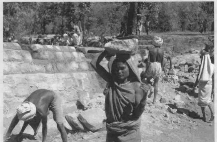
Village woman working on a diversion project.
