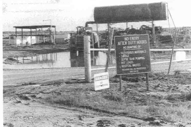
The raging Salt River washed away one-third of the Tri-Cities Landfill on the Salt River Pima-Maricopa Indian reservation east of Phoenix. (Photo: Barbara Tellman)
