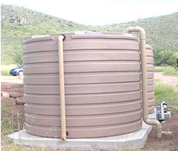
Figure 9. Two 2825-gallon cisterns installed in the foothills of the Huachuca Mountains, AZ. Photo courtesy of Mary Ann Capehart.
