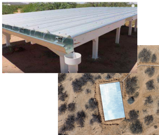
Figure 8. Two rain roofs in southeastern Arizona made with recycled materials. Photo (top) courtesy of Joe Mooney, Homesteadonomics You Tube channel. Photo (bottom) courtesy of Derek Howlett, Handeeman You Tube channel.
