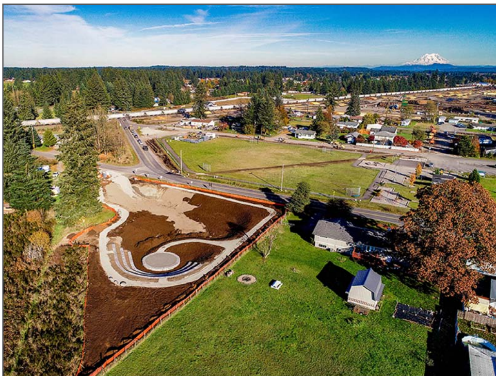
Albany Street Stormwater Pond, Rochester
