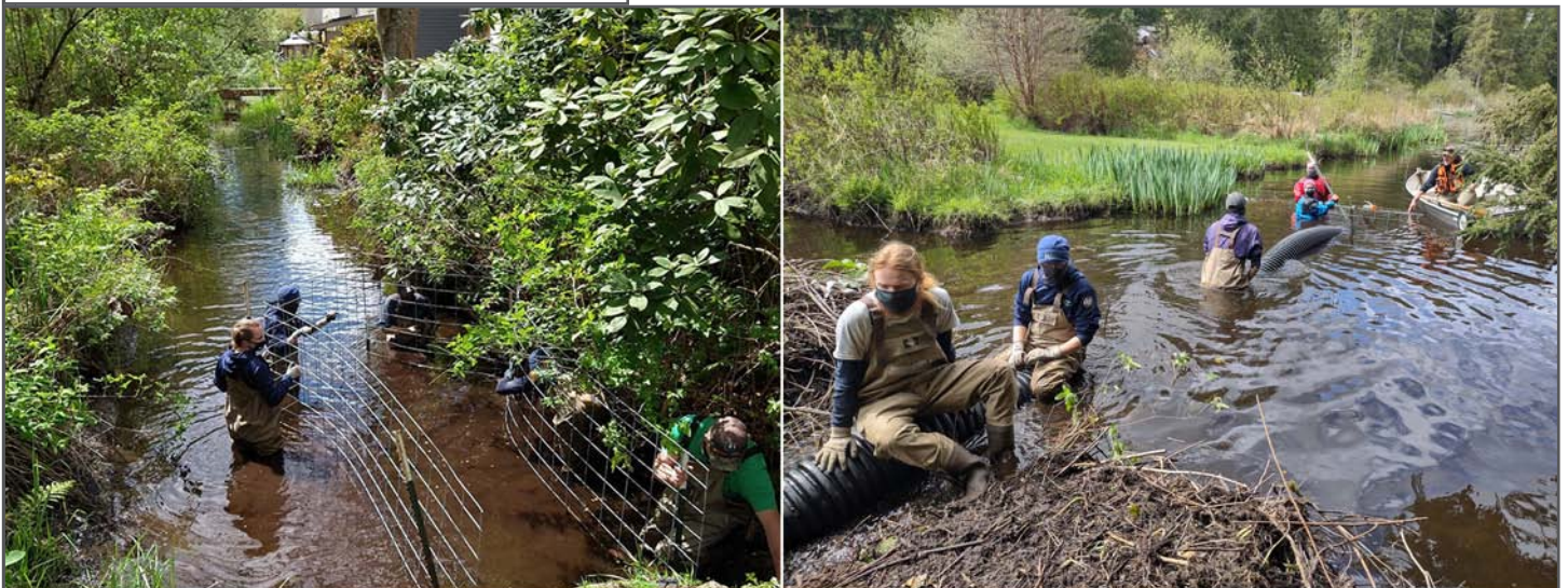
Beaver Coexistence: Fencing & Pond Leveler Installation - Photos by Snohomish Conservation District
