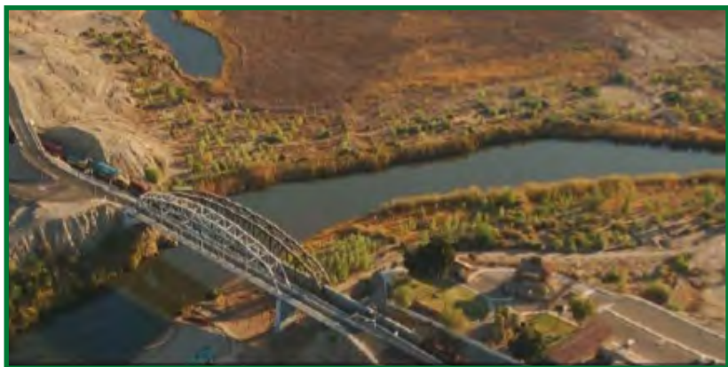
Aerial photo of Yuma Wetlands. Photo courtesy of Fred Phillips.
