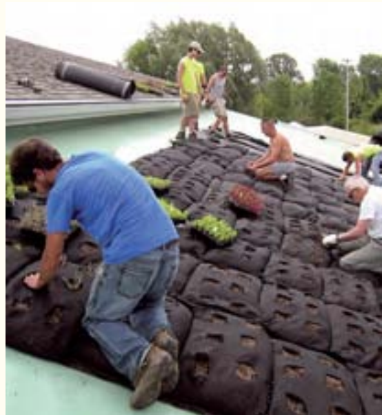
Milwaukee Metropolitan Sewerage District
