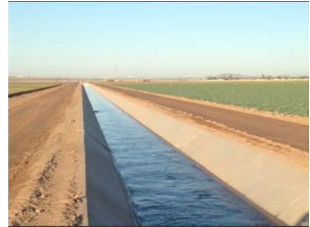
Concrete Lined Canal
